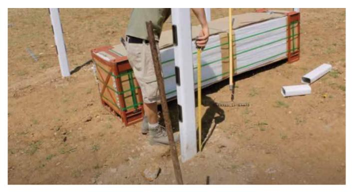
5. Set the post to a height of 57" from the ground. Run a string line along the planned fence line at the same 57" height to ensure all posts are set to the same height. Keep in mind the ground will vary a few inches up and down even on a relatively flat terrain. You want the fence line to look very straight where the terrain allows and with very gradual undulations in varying terrain.
