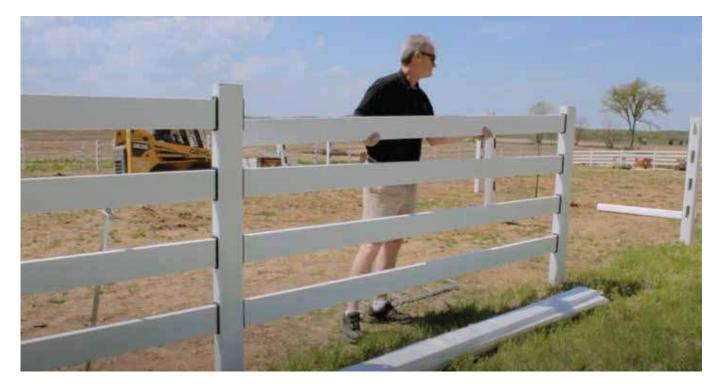
3. Starting at a gate or other terminal post (post #1), insert one end of the rail into the top rail opening on the next post (post #2) all the way until it bumps the back side of the post and then swing it into position and insert the other end back into the top rail opening on post #1.
