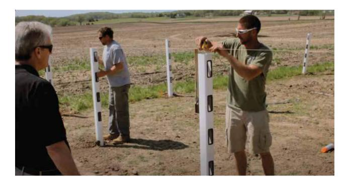
6. Pour concrete up to 2-4" below ground level. Work concrete into hole by shaking post. Use post level to ensure the post is plumb and in line and not rotated out of square. After the concrete is set, fill the rest of the hole with dirt.
