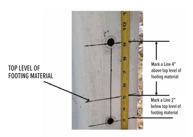
Drill one ½" hole on each marked line(4" above top level of footing material and 2" below top level of footing material), it is recommended that you use a step drill. Each hole should be drilled approximately on center of the post face (2 9/16" from the edge of the post) it is okay if the drill walks off the line you measured as the mounting holes are slotted to provide minor adjustments. Once the holes are drilled, insert the rubber well nuts as shown in the picture below.
