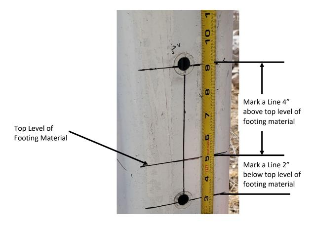
2. Drill one ½" hole on each marked line(4" above top level of footing material and 2" below top level of footing material), it is recommended that you use a step drill. Each hole should be drilled approximately on center of the post face (2 9/16" from the edge of the post) it is okay if the drill walks off the line you measured as the mounting holes are slotted to provide minor adjustments. Once the holes are drilled, insert the rubber well nuts as shown in the picture below.
