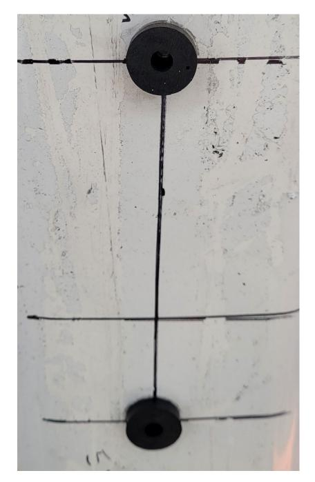
3. Place the mounting backet over the well nuts and inset one of the screws into the top slotted hole and screw into the well nut, do not tighten down fully.
