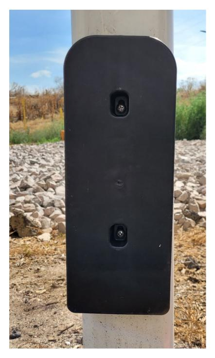
5. Insert rails into bracket from the top, two rails per side. End posts will only use one side of the bracket.
